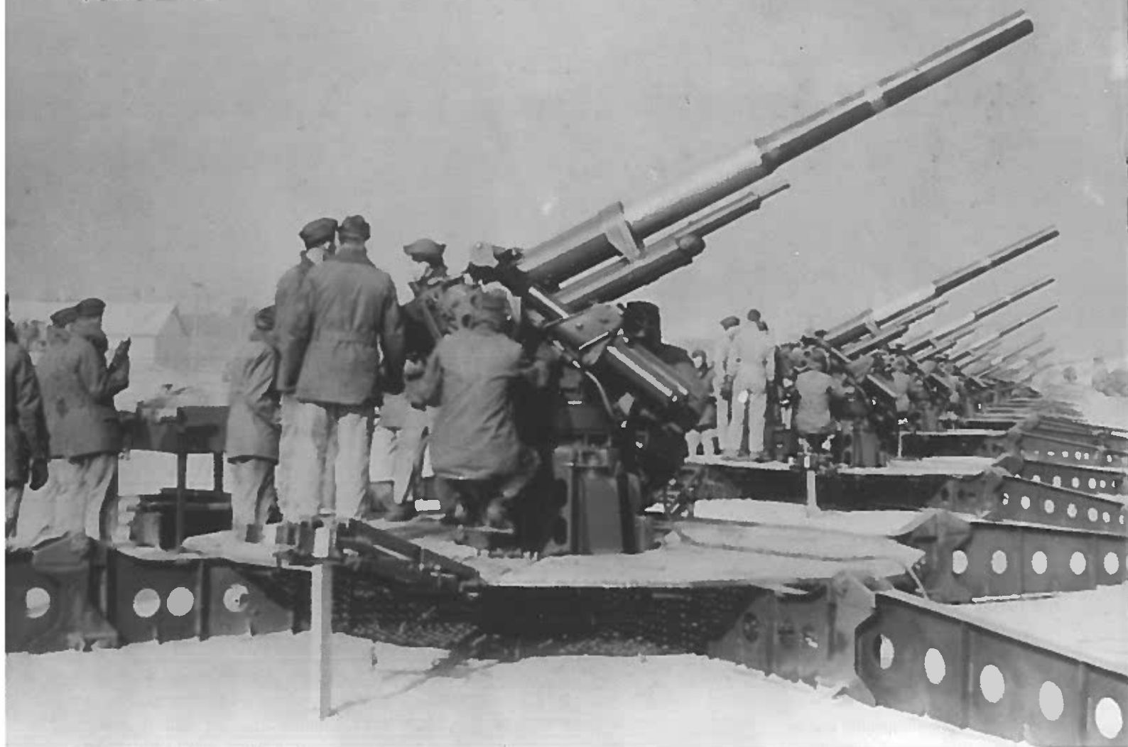
Gunners of the 71st Coast Artillery Regiment (Antiaircraft) train on M3 3-inch antiaircraft guns at Fort Story, Virginia. The M3 became the Army's standard AAA piece in 1928. (National Archives)
